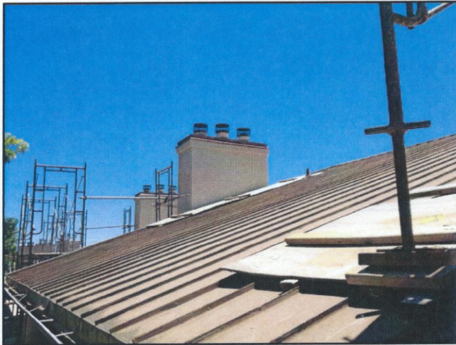
Views of chimney veneer repairs. New flashing at the top has been installed. EIFS veneer application is in progress.
