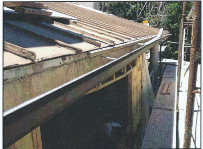
Views of roof eave drip line and gutter. This flashing metal was found to be in very poor condition. The drip flashing will be replaced and new gutter straps will be installed.
