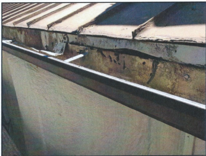
Views of roof eave drip line and gutter. This flashing metal was found to be in very poor condition. The drip flashing will be replaced and new gutter straps will be installed.
